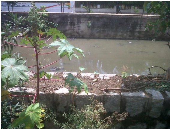
View of Storm Water Drain at Wilson Garden
