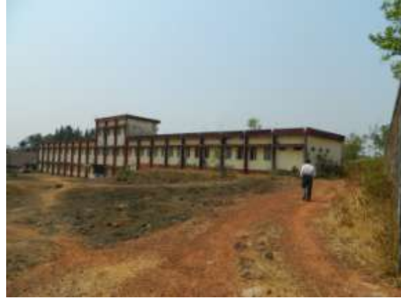
Existing Structure Present at the Site
