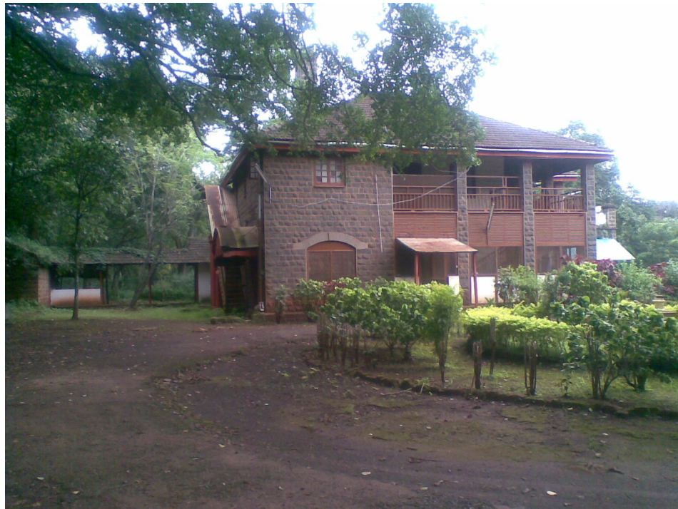
Figure 3: Existing building at Vaccine Depot
