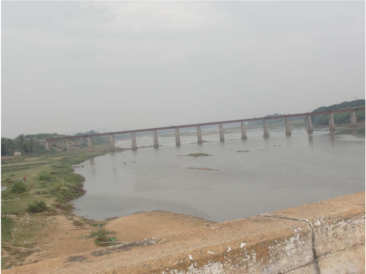
Fig 3.4: Photograph showing the River Tungbhadra flowing near the proposed project site
