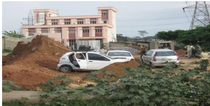
BESCOM Construction on Project Site
