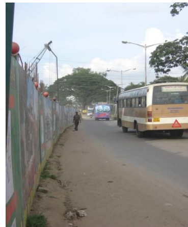
Road In front of Metro Station site
