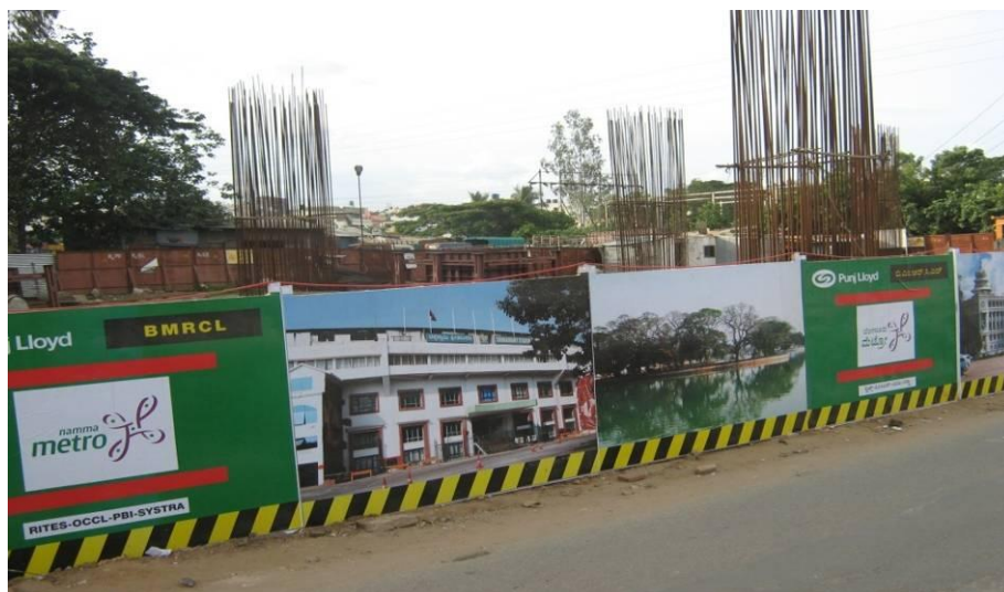
Metro Station construction in front of the project sight
