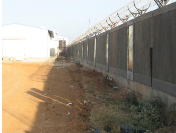
Figure 5 View of the BMRCL Yard Boundary Wall
