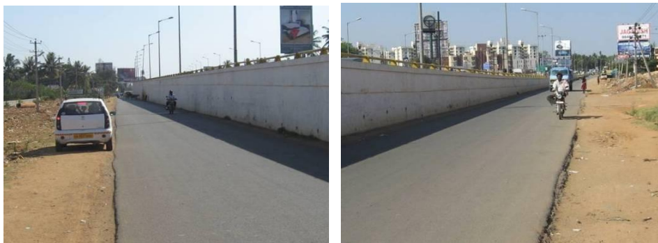
Figure 12: Service road adjacent to the Yelahanka bypass
