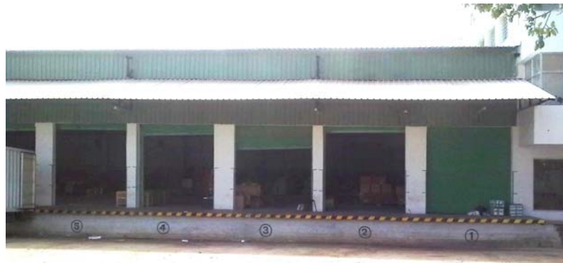
Figure 35 Safexpress Facility – Docks (Numbered & Leveled)
